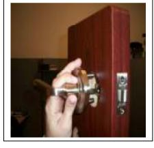
→ 5) Insert the remaining lock-half into the public (outside) side of the door. Note that the two threaded mounts on this lock-half insert into the larger tubes on the other lock-half.
