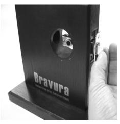
→2a) Insert latch mechanism into door. If using a <u>privacy</u> latch, make certain the threaded button is facing the side of the door from which you wish to lock the door (inside/non-public) Dril
